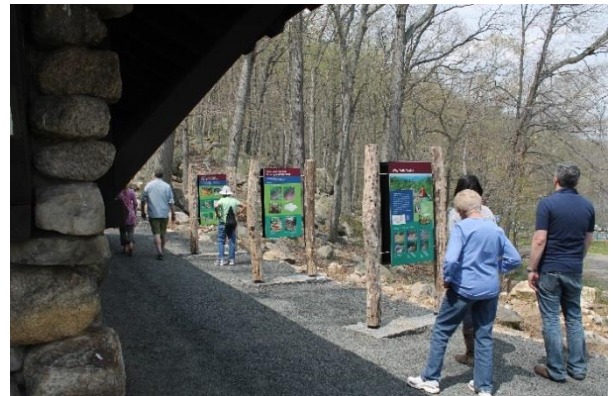
To solve overuse and misuse issues on trails at Bear Mountain, the Trail Conference has rebuilt and restored the Appalachian Trail—including the construction of an accessible section of the Trail—and built an interpretive trailside exhibit, both part of the multifaceted Bear Mountain Trails Project. (Photo credit: Jeremy Apgar; Amber Ray)
